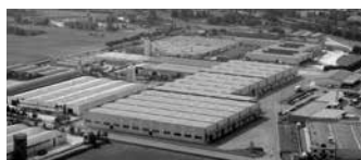
San Giovanni al Natisone (Udine, Italy) Assemblaggio tavoli e sedie, magazzino Tables and chairs assembly lines and warehouse 40.000 sqm
